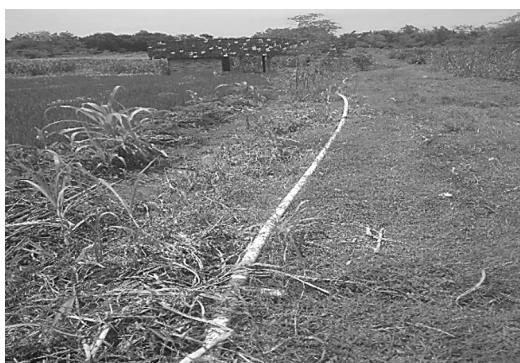
Fig. 8. Installation of valves and distribution networks.
