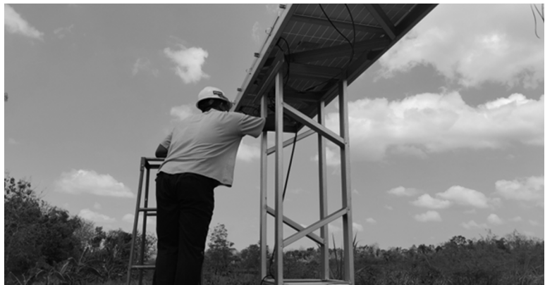
Fig. 6. Setting up solar panels with parallel circuits.
