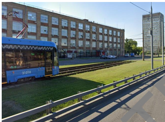
Fig. 3. Location of streetcar tracks away from the carriageway (Google Maps image source: https://maps.app.goo.gl/hboT7FKguRLMihR59 )
