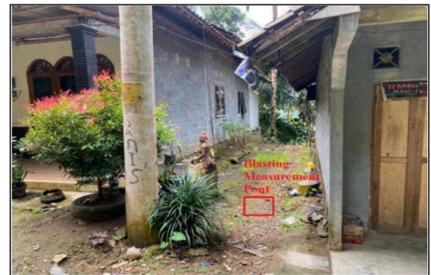
Fig. 6. Ground vibration measurement point.
