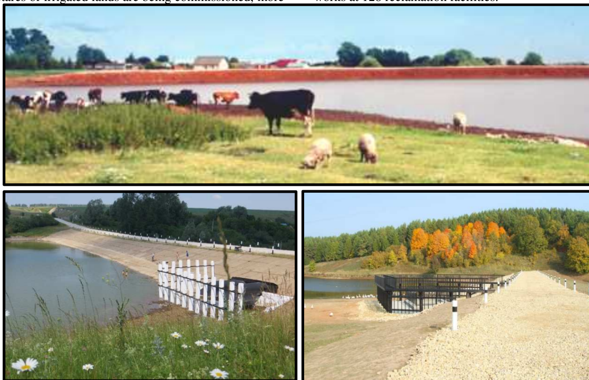
Fig. 2. Restored hydraulic structures in the Republic of Tatarstan
