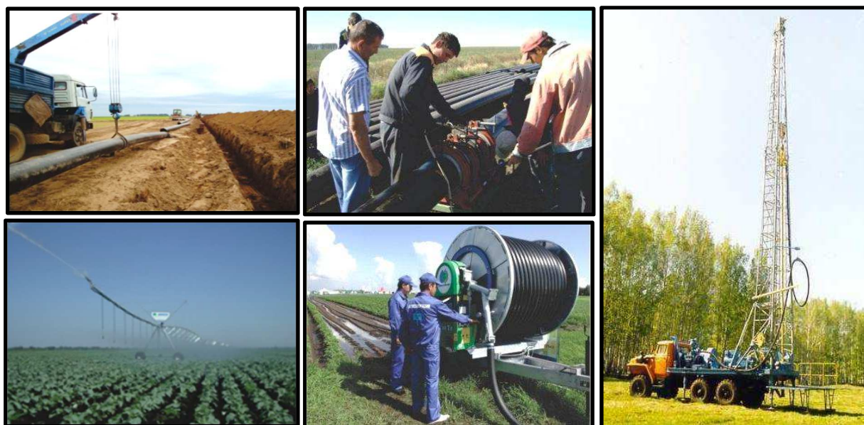
Fig. 1. Construction of infrastructure facilities for amelioration
