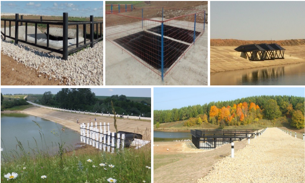
Fig. 1. Hydraulic structures in the Republic of Tatarstan.
