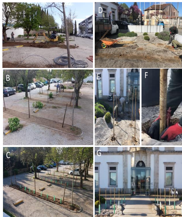
Figure 3. Main phases carry out during urban vineyard implementation in 2019 for car park (A to C) and in front of the main hotel entrance (D to G). Photos from authors.
