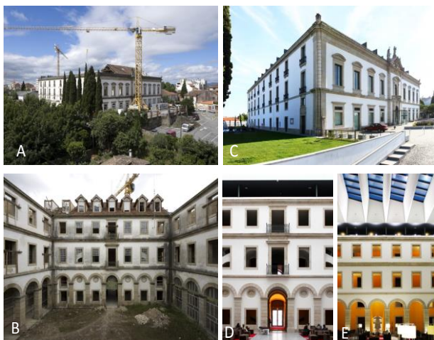
Figure 1. Overview of the Hospital's conversion works (A and B) and final appearance of the entire building of the Historic Hotel in 2009 (C, D and E). Photos from Santos [3].
