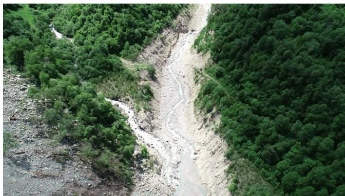
Fig 1. Landslide-flow near the village of Dachu-Borzoy
