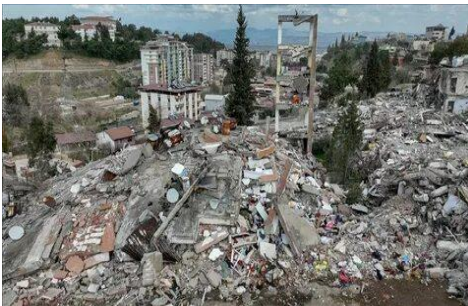
Fig. 2. Earthquake in Turkey 06.02.2023
