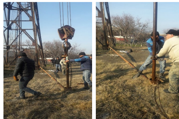
Fig. 1. The current condition of the submersible water pump, which provides drinking water to the population of Khavos district of Syrdarya region, has become unusable today.
