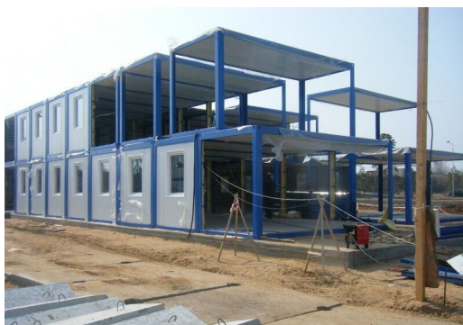
Fig. 1. Installation of temporary modular buildings.
