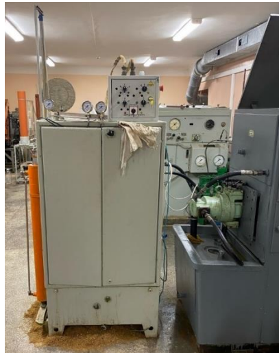
Fig. 1. General view of the test bench for testing choke flow dividers/adders
