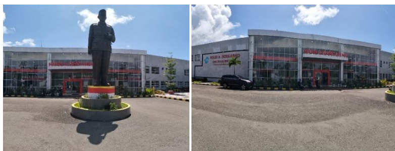
Fig. 9. Health facilities at Soekarno Morotai Hospital
