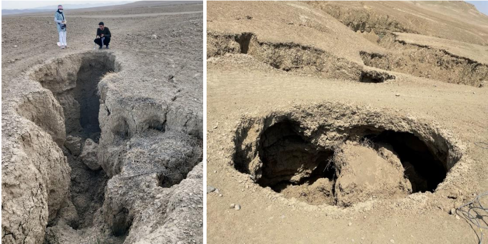
Fig. 2. The examples of collapsed calvities in the study area.
