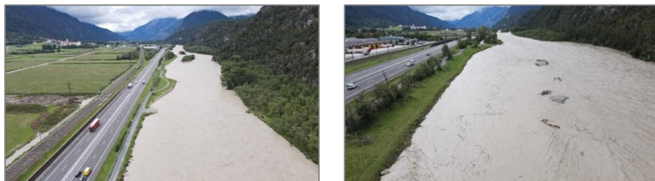
Fig. 4. 100-year flood on 28.08.2023
