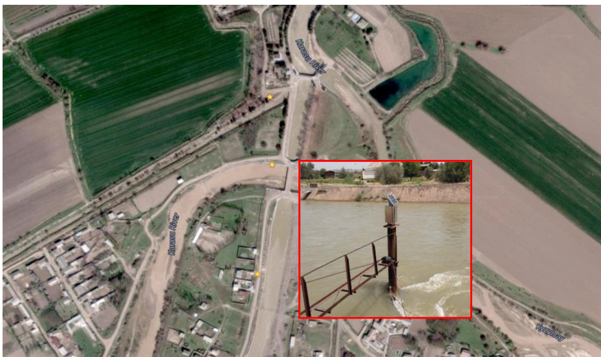
Fig. 6. The installation of automatic flow meter.
