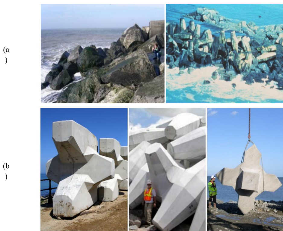
Fig. 4. Illustrations of Armour Units: (a) Damaged Cube (Left) and Dolos (Right), (b) Accropode (Left), Core-loc (Middle), and Xbloc (Right) [11]
